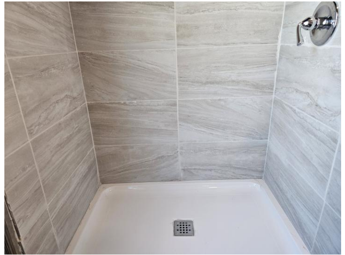
New shower installed in upstairs bathroom
