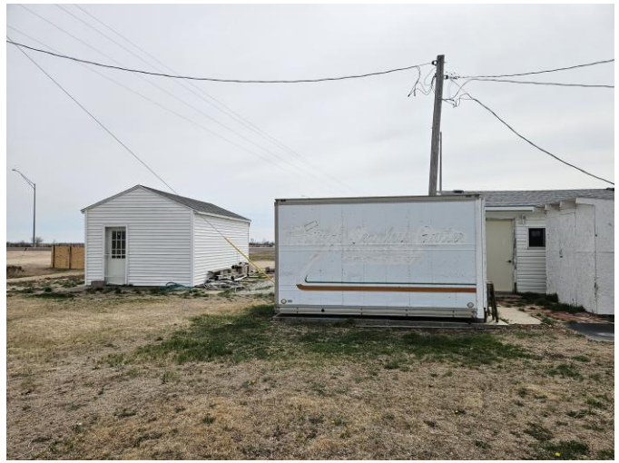
Storage container and East end of smokehouse
