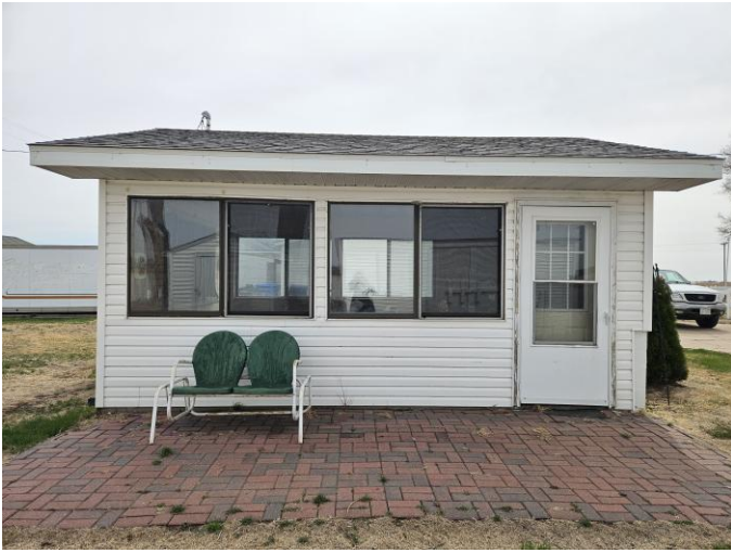
Potting Shed – Former hot tub room
