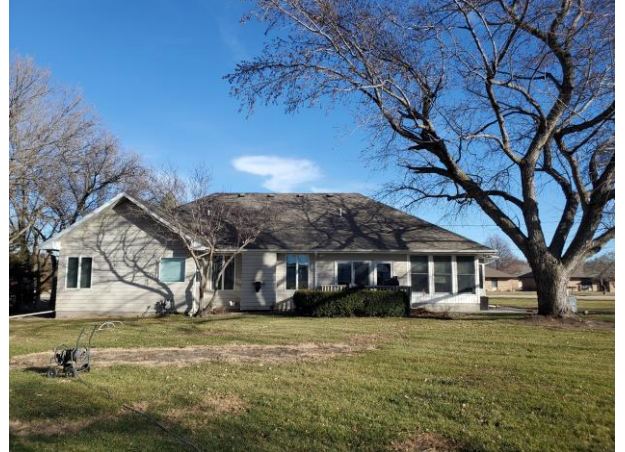
West side of house
