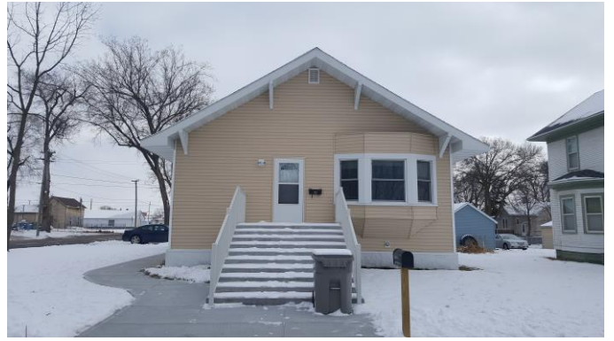
New front steps and concrete
