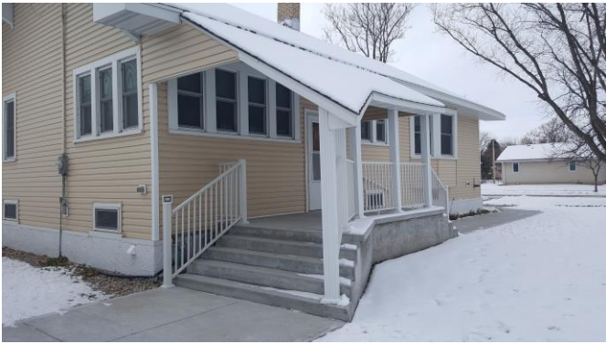
New East steps and concrete
