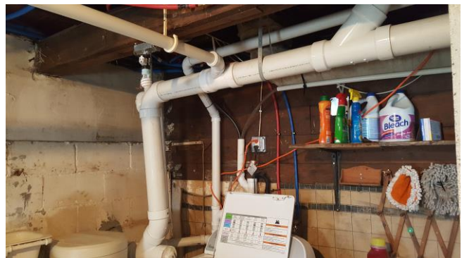
New plumbing in basement
