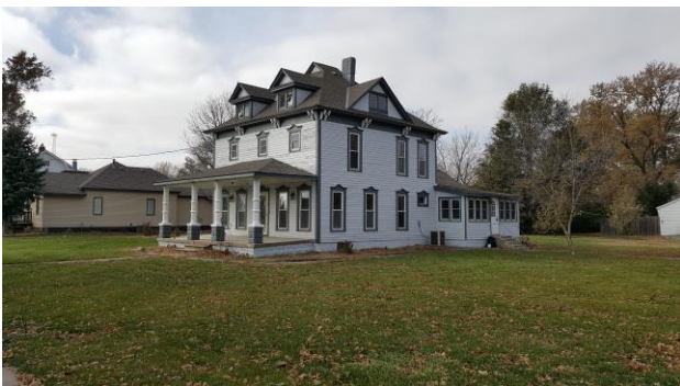
View from East side
