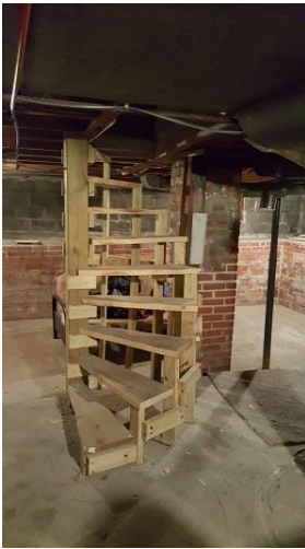
New stairs to basement
