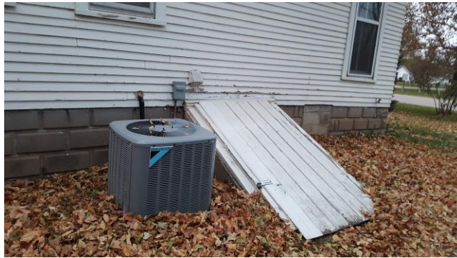
New central air and new Cellar door
