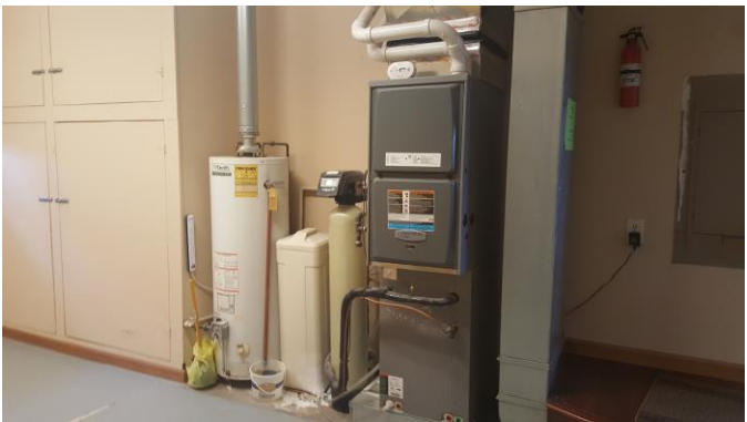
Mechanical room/Storage area
