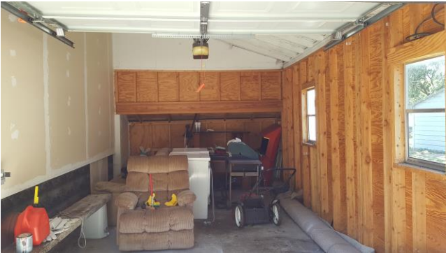
Attached 1 car garage
