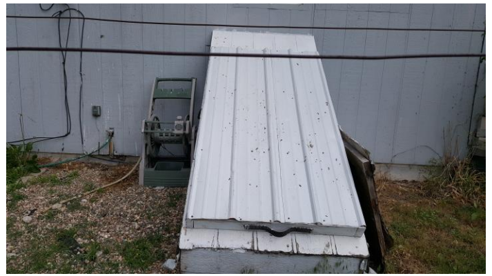
Exterior door to basement area
