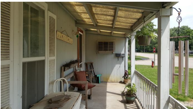
Front porch showing window air conditioner
