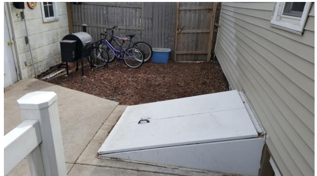
New door into crawlspace & concrete patio
