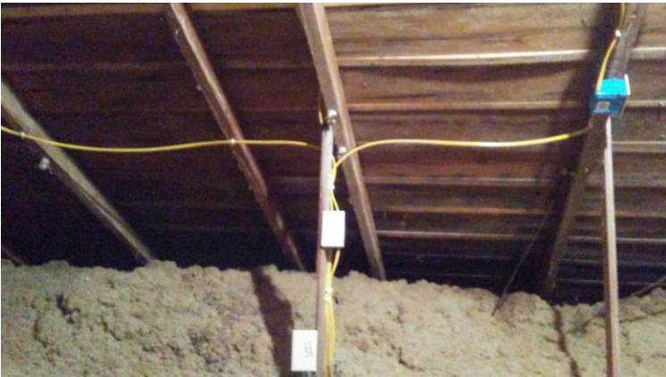
Attic showing new wiring and insulation
